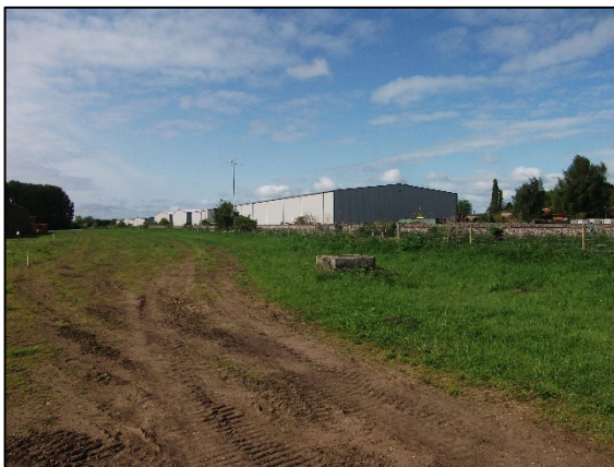
View along western site boundary with adjacent (raised) railway line and industrial buildings beyond
