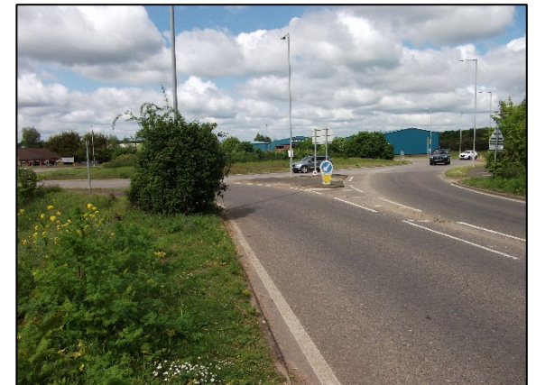
Junction of A17 slip road and industrial estate roundabout
